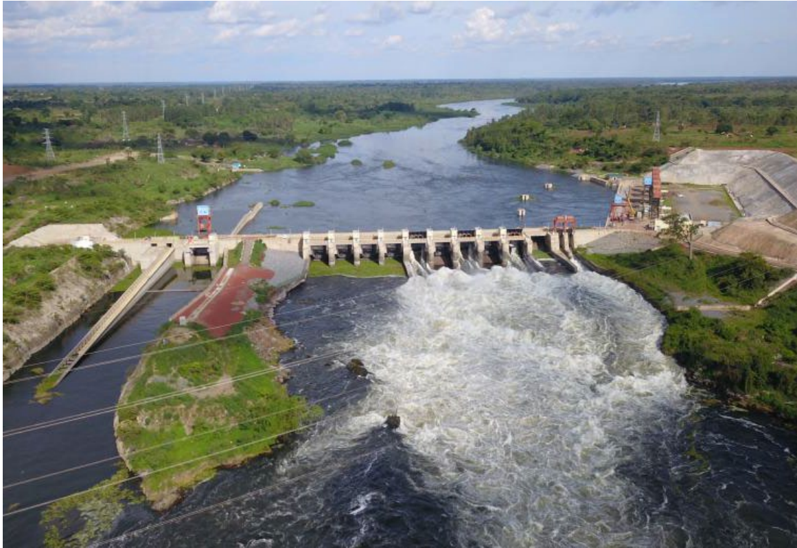
Figure 1-3 Karuma Hydropower Station
