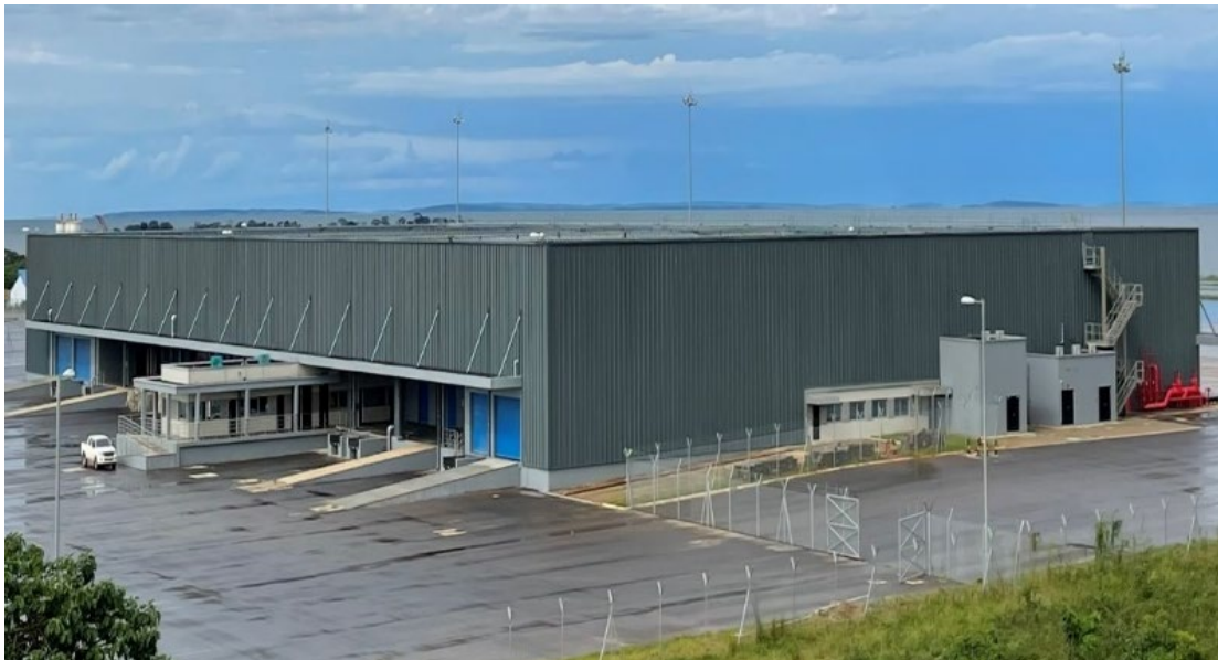
Figure 1-6 The Upgrading and Expansion of Entebbe International Airport Project
