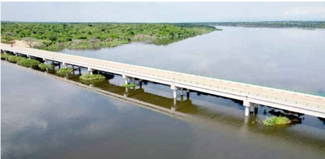
Figure 1-15 Paraa Bridge Built by Chinese Enterprises in Paraa National Park
