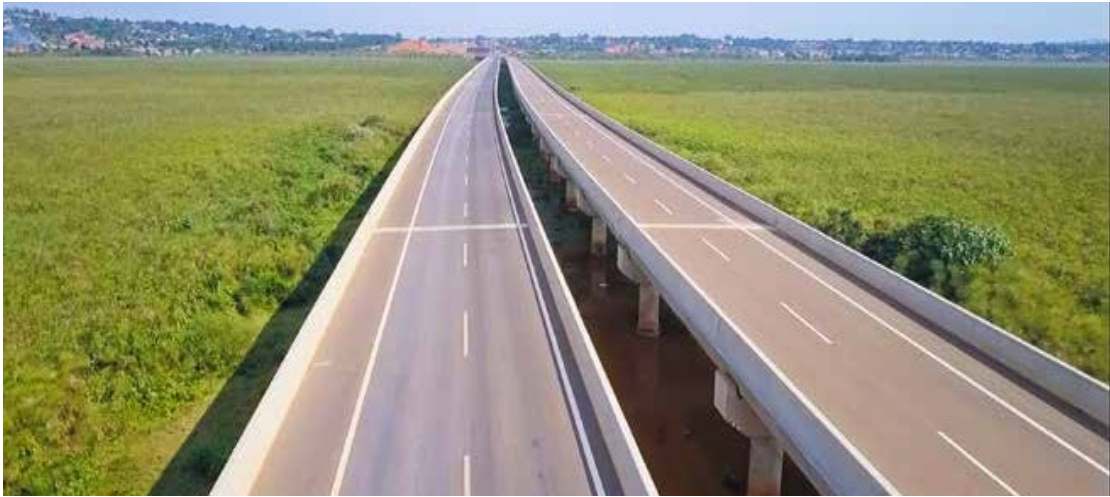
Figure 1-14 The Nambigirwa Bridge Built by Chinese Enterprises in the Swamp
