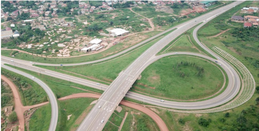
Figure 1-5 Kampala Entebbe Expressway
